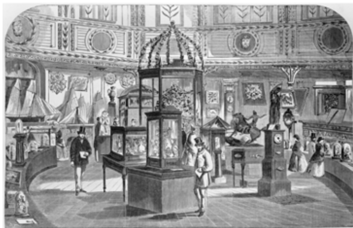
The Intercolonial Exhibition: interior of the rotunda State Library of Victoria
